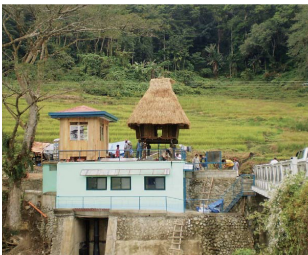
© Global Sustainable Electricity Partnership. Mini-hydro plant.
